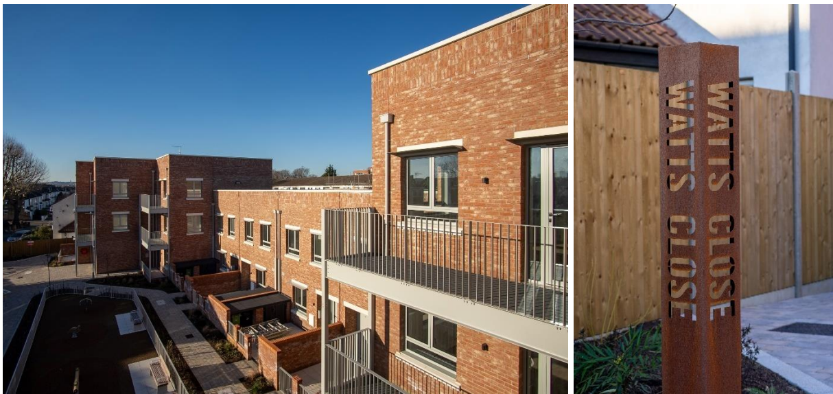
Figure 10: Aerial view of development with 16 new apartments accessed of Watts Close and two new houses accessed off Lomond Close. Photograph of the Watts Close signage.
